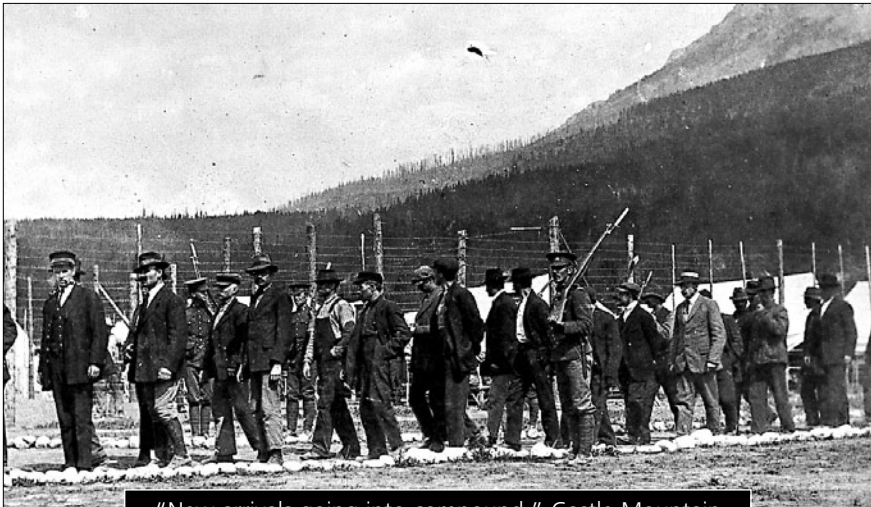
“New arrivals going into compound,” Castle Mountain
