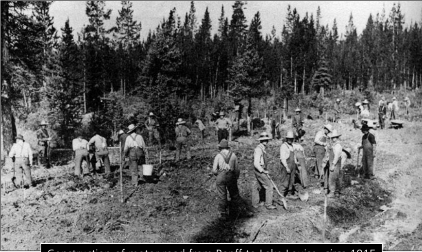
Construction of motor road from Banff to Lake Louise, circa 1915
