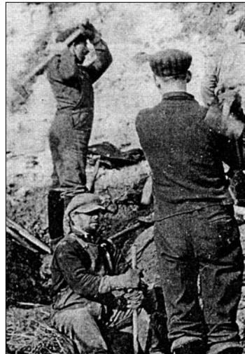
Internee construction crew near Edgewood, British Columbia
