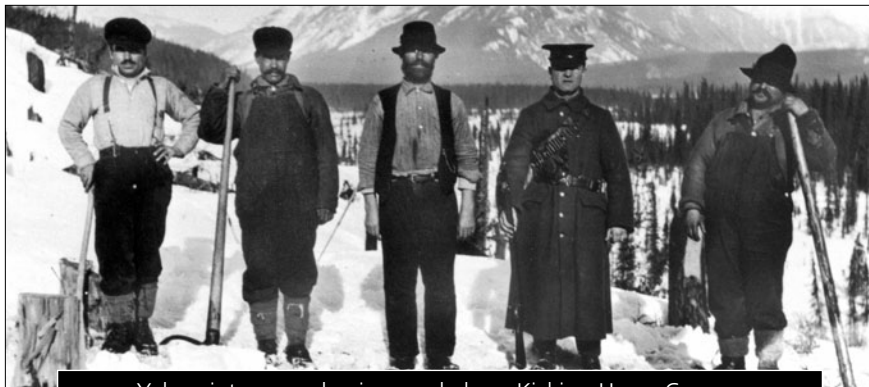
Yohoo internees clearing road along Kicking Horse Canyon
