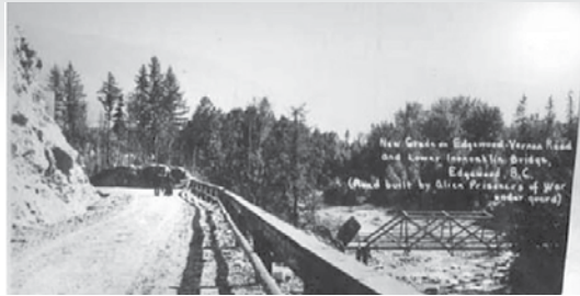
Hwy 6 Vernon Edgewood road and bridge construction, Arrow Lake Historical Society photo
