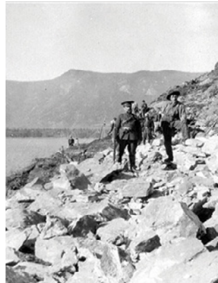
Hwy 97 Construction at Mara Lake, Royal BC Museum Archives photo E - 89149
