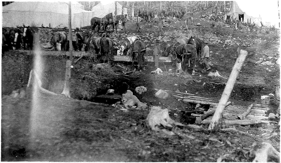
Contractor's camp and teams.
