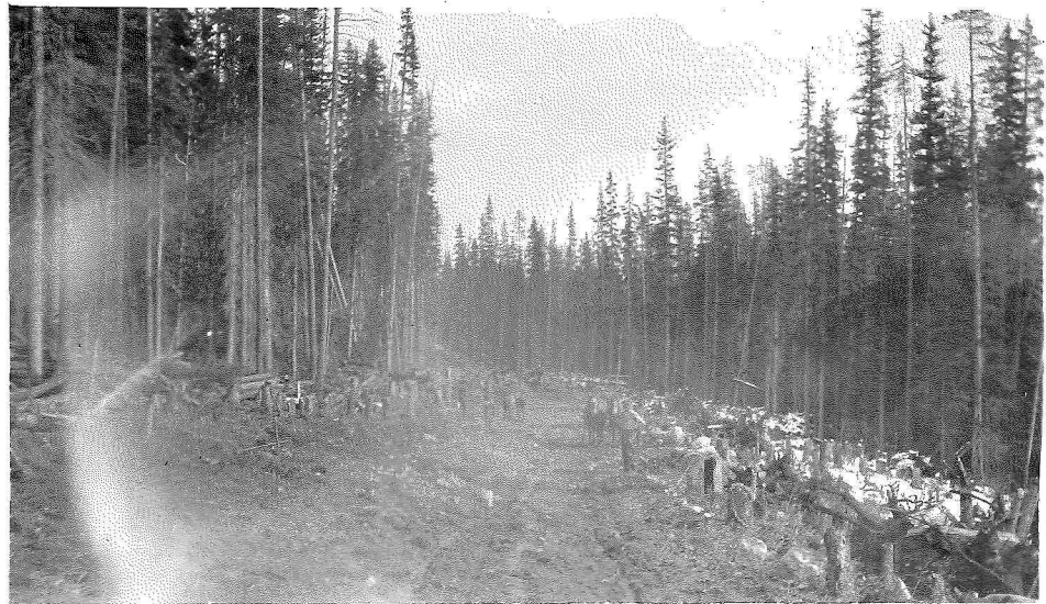
Part of Grading, - Sta. 212.
