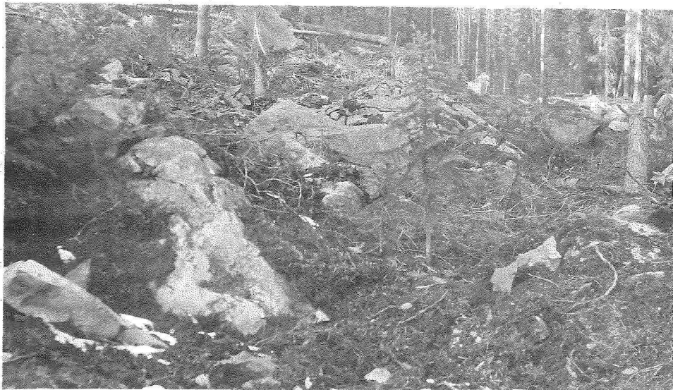
Sta. 475.- after clearing
