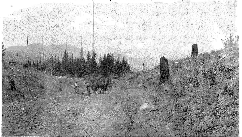
Construction at Sta. 117- Section 4
