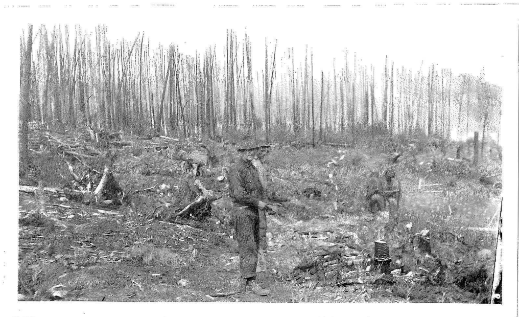
Construction, near Sta. 186.
