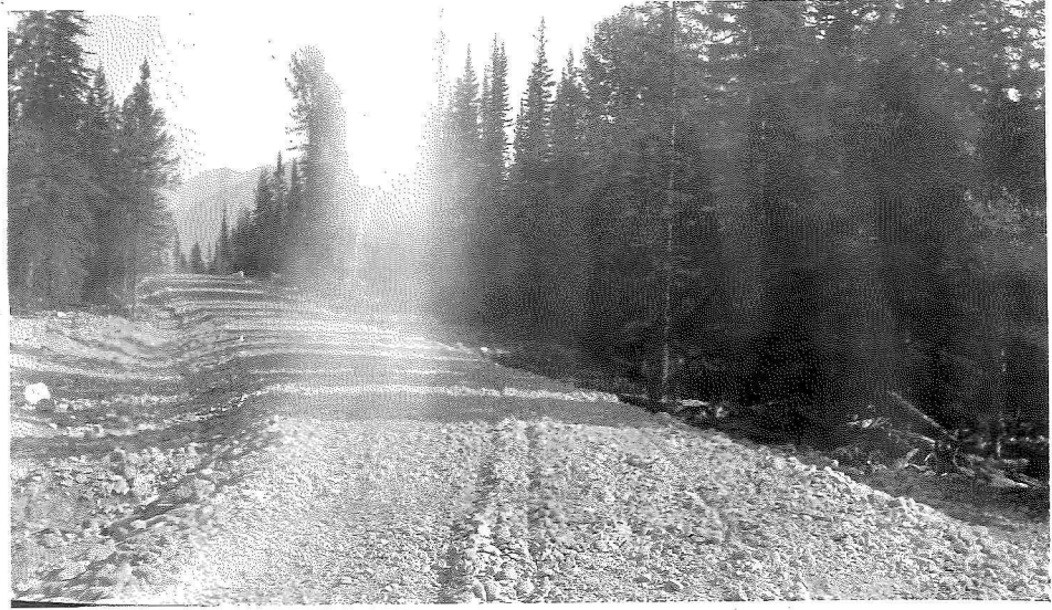
Road over Rock Wash - Sta. 296
