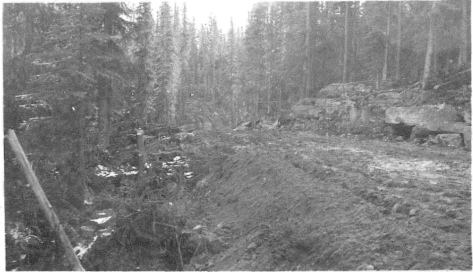
Sta. 450.- during Construction
