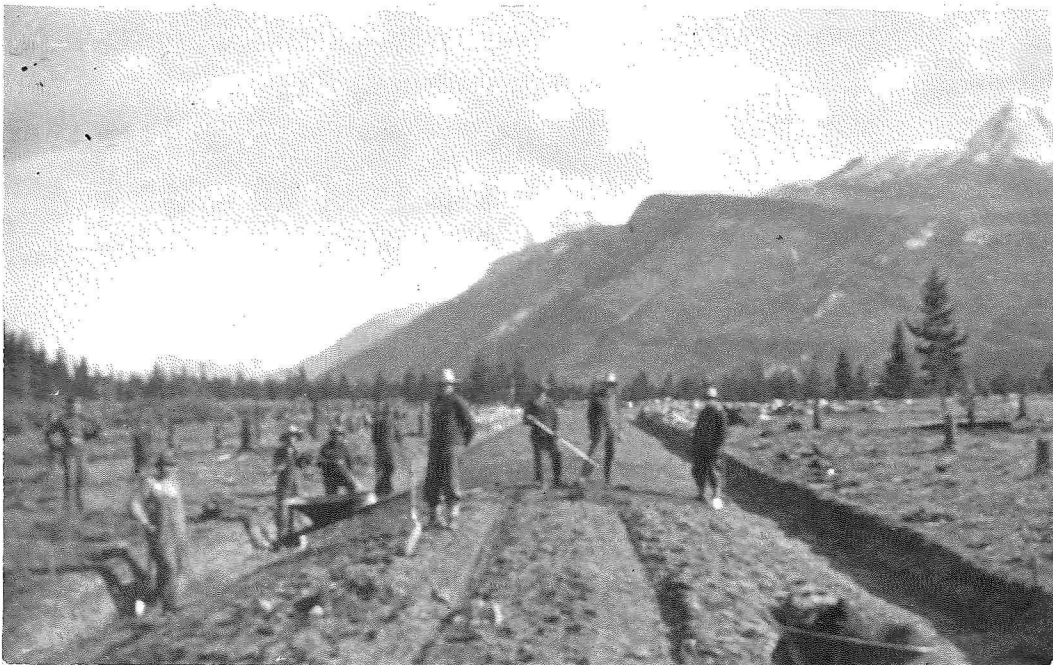
Finishing sub-grade - Castle-Laggan road.
