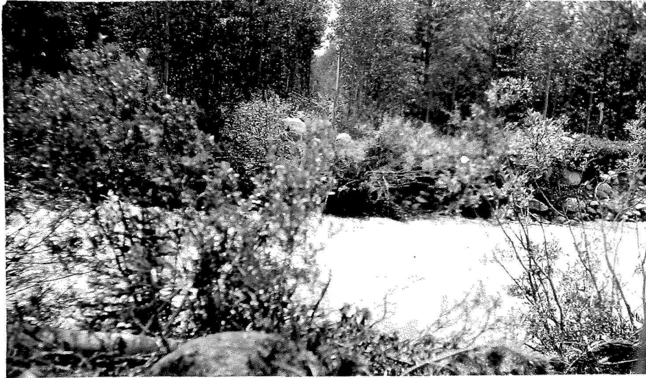
Bridge Site - Sta. 500 Baker Creek
