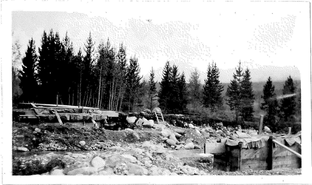
Concrete in forms - Baker Creek Bridge piers - Sta. 500
