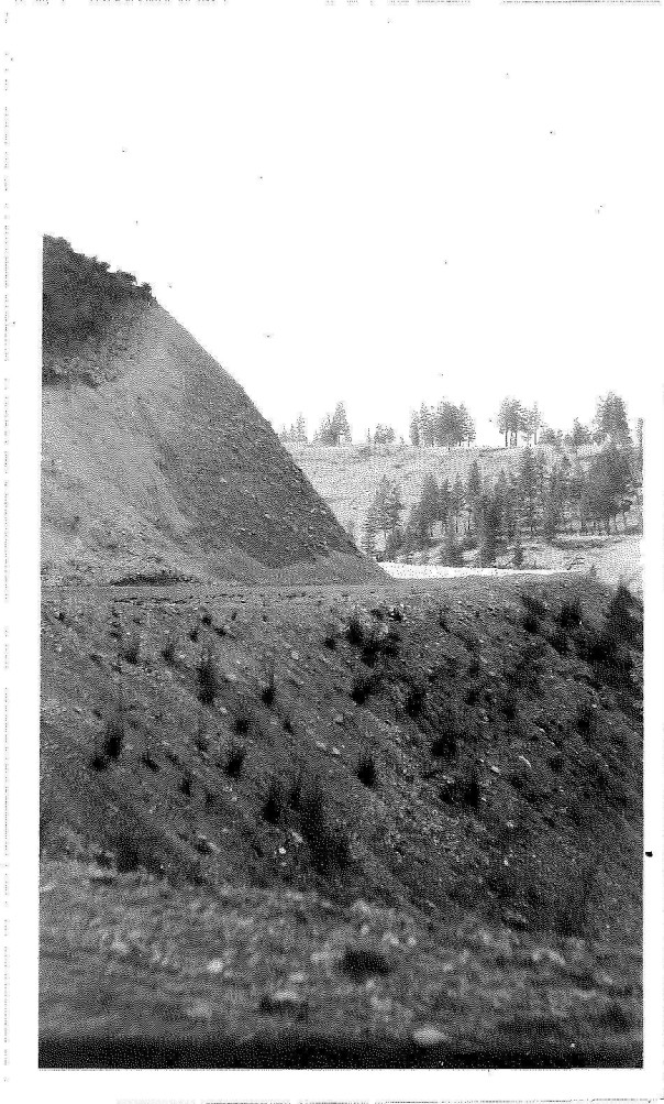
Sidehill cut on Sinclair Road.
