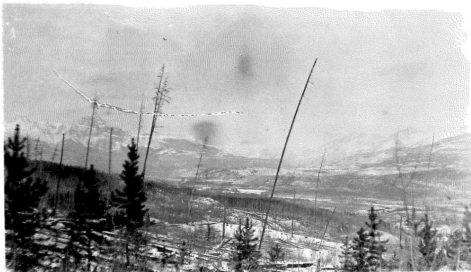
Looking North from Sta. 502 - Mt. Edith Cavell Location Line.
